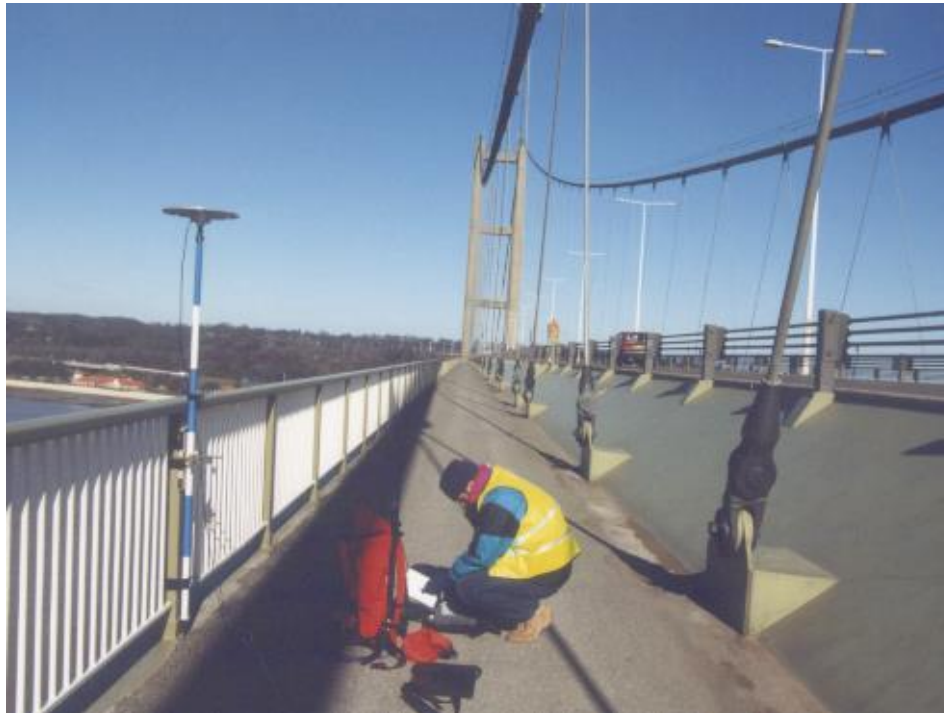
Figure 4 - The GPS receiver located at the mid span
